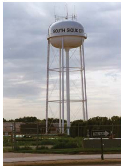
South Sioux City Water Storage Tower, 2000 Photo.
