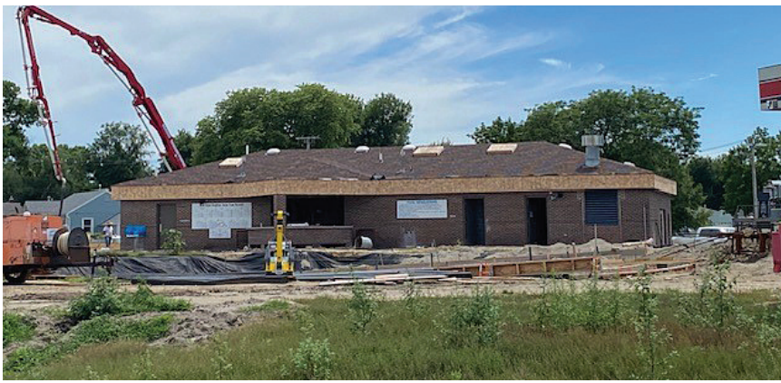
Crews pour concrete for the lower walls of the equipment and chemical feed building for the new pool in West Point. The adjacent building is the original bathhouse that is being remodeled and restrooms are being added to the west end of the bathhouse that will be available year-round to accommodate all the activity in Neligh Park. Photo shared courtesy of the City of West Point
