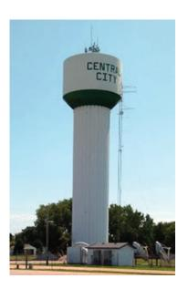
**The water tower** was completed in January 1974. It holds 500,000 gallons of water and is 160 feet tall.
