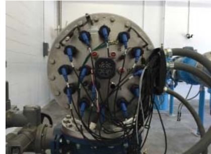
UV disinfection chambers
