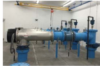
UV disinfection piping
